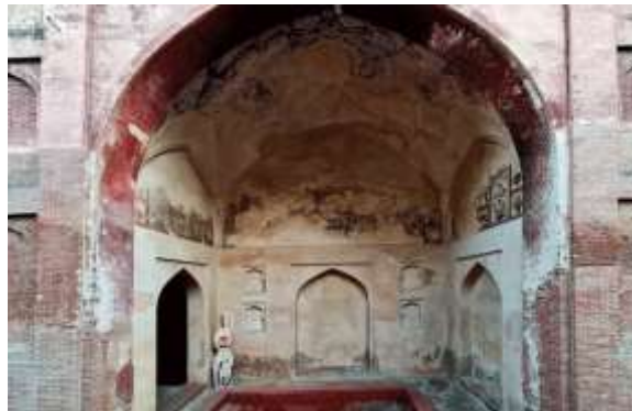
Figure 2 Entrance Door Shahi Hammam Lahore, Current Condition
