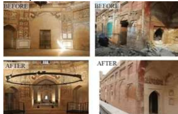
Figure 1 Before and After Image from "Restoration and Conservation of Shahi Hammam"
