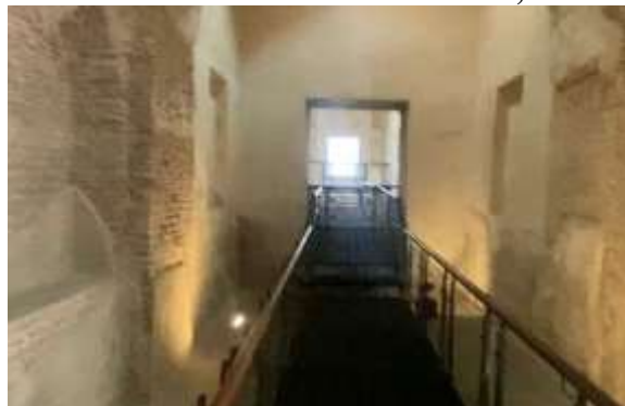
Figure 3 Corridor towards the Entrance, Current Condition
