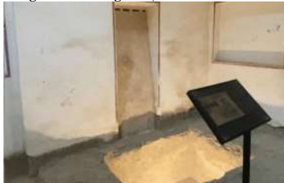
Figure 6 Cold Bath, Current Condition
